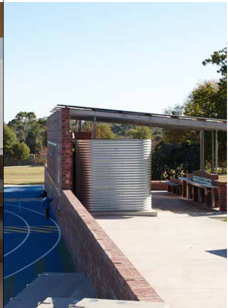
Figure 7: Box Hill Gardens, NMBW Architecture Studio and Aspect Studios, 2013: Hit-up wall and shared handbasins.
